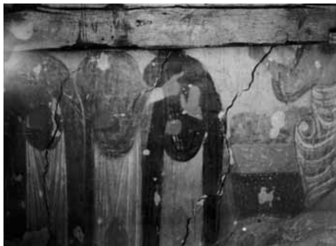
Photo from Fornåsa parish archive showing the beam in the roof construction that was added in 1900 and hiding parts of the murals until 1954 as it became removed
