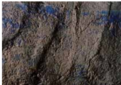
The surface character of the intonaco: traces after tool marks from the smoothing process of the intonaco (photo A. Henningsson)
