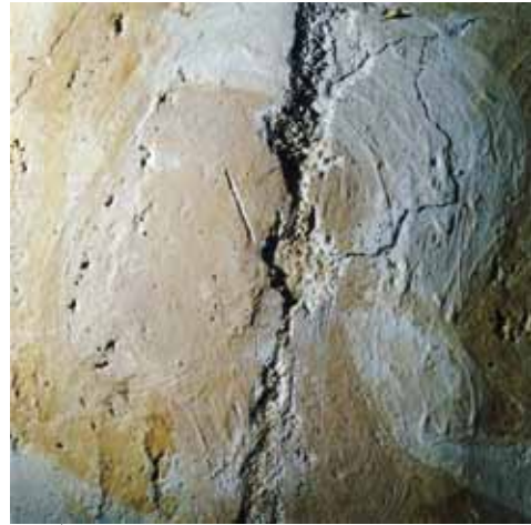
Through lacunas in the 2 mm thick intonaco an arriccio of 8 mm can be seen. Further a 1 mm thick lime wash layer is applied to the arriccio (photo A. Henningsson)
