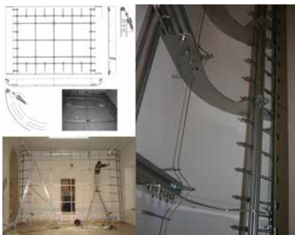
Fig.8 : Stretcher design and assembling (Photo © Artbee Conservation)
