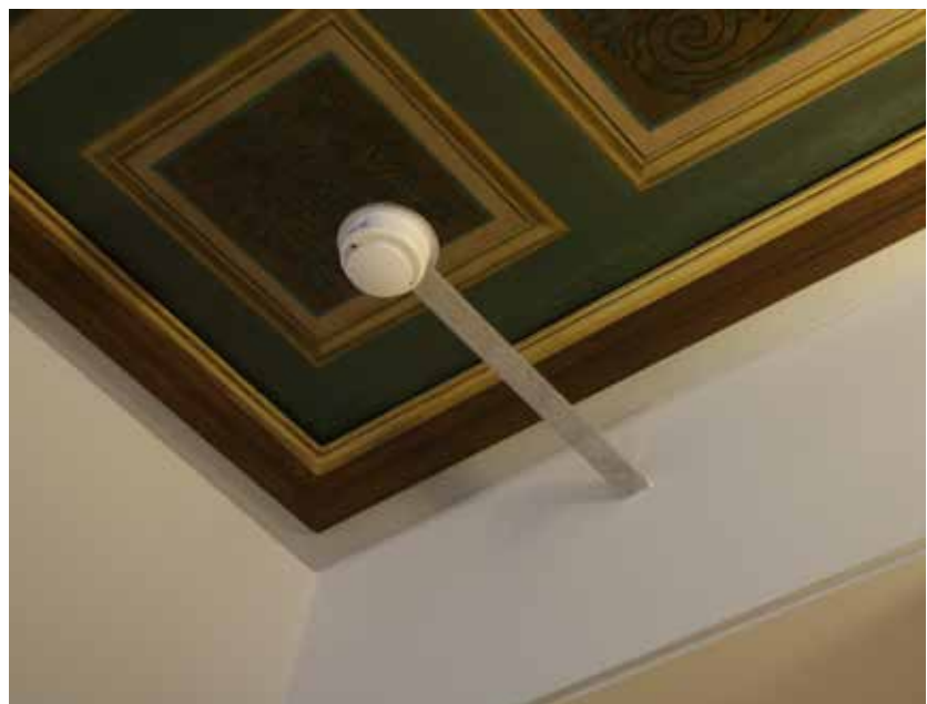
Fig. 18 : A fire detector attached to the side wall (Photo © Artbee Conservation)
