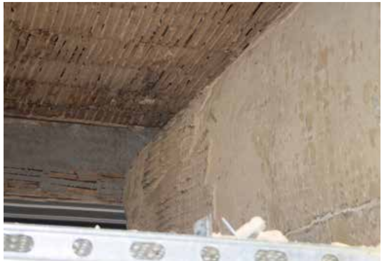
Fig.14 : During the removal of the mortar (Photo © Artbee Conservation)
